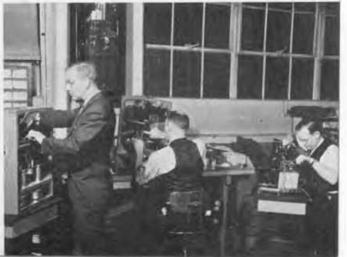
One of the jobs of the winding and transformer assembly department is to produce Variacs. C. W. Whitehead (left) operates the machine winding a TYPE 50 Variac. At the right is R. W. Searle, foreman.
